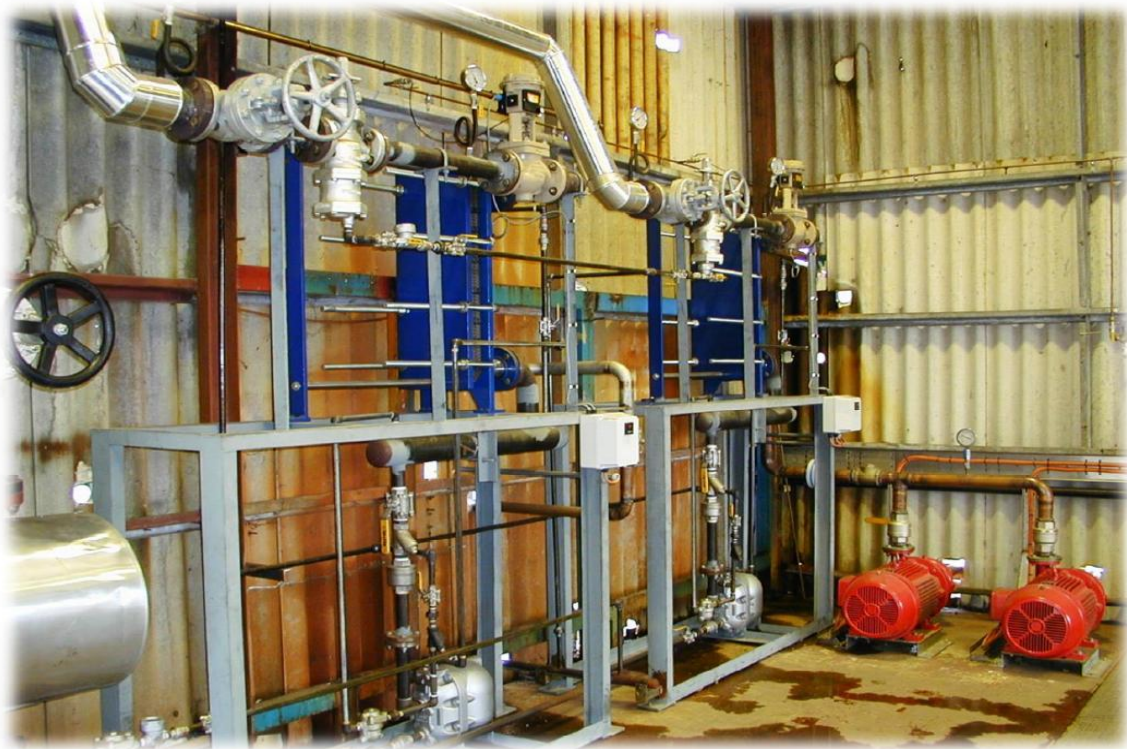
Installation with steam / condensate trap
